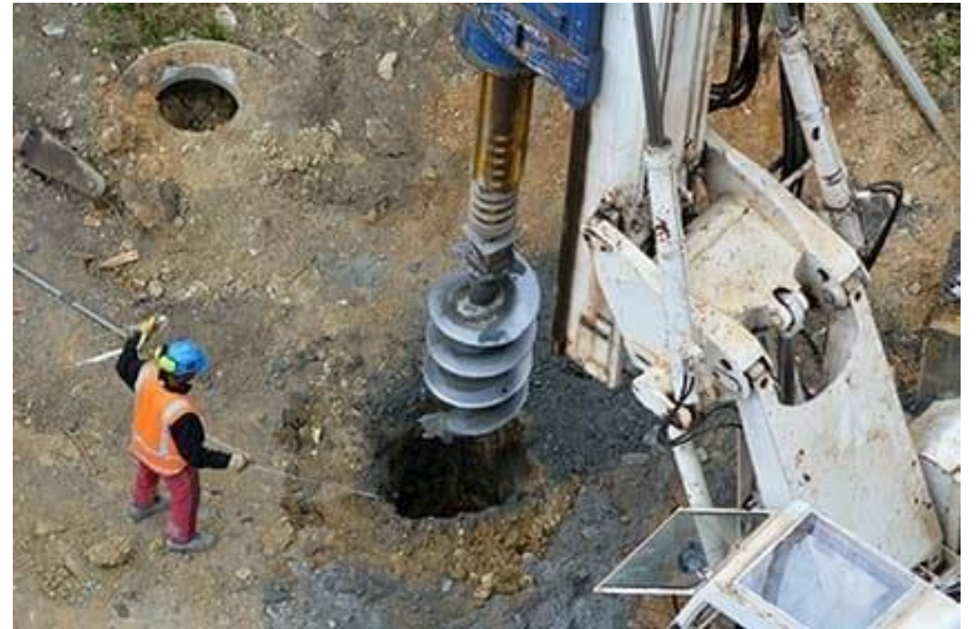
Drilling & Pile Driving
